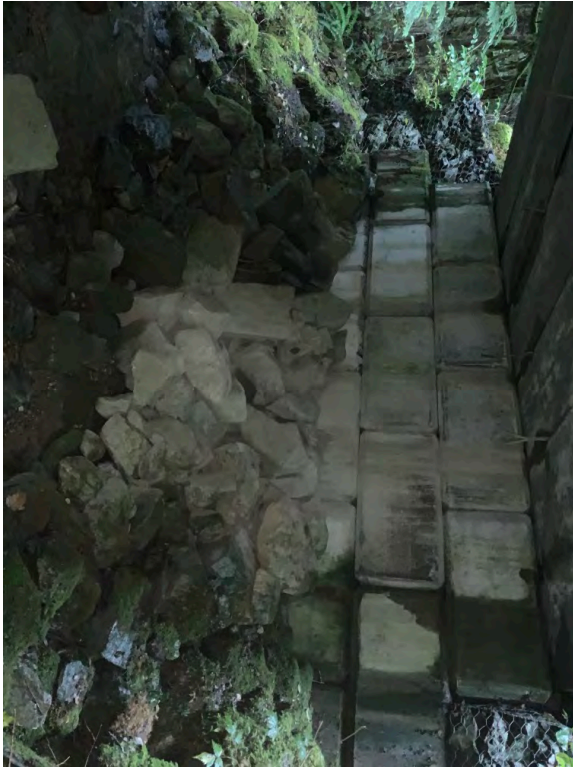
Right Bank Abutment when facing downstream
